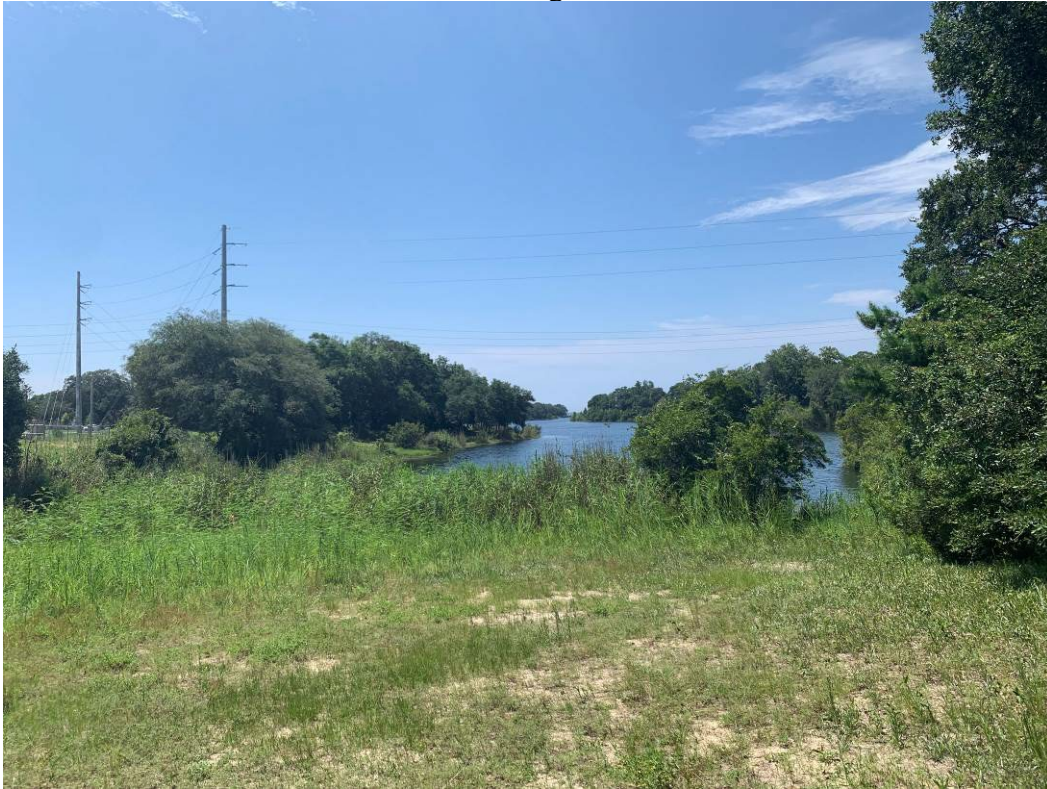
Picture 21. OSW B looking south from dam area.
